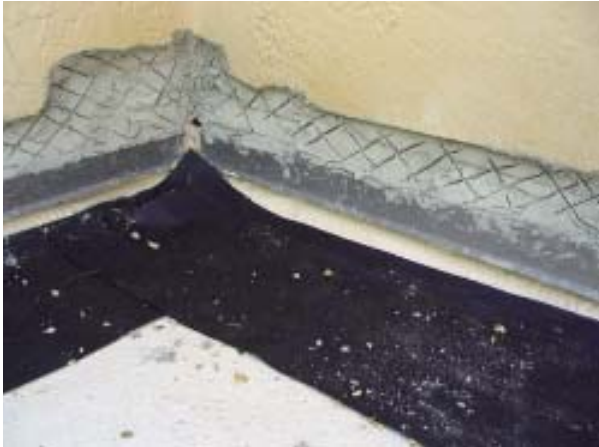
Figure 5. Foam is self-flashing when applied to waterproof substrates, but water can still get behind wall cladding. Therefore, the crew breaks out this stucco, slips counterflashing behind the building paper, and laps it over the foam below (above). Where the foam runs up onto the wall, the roofer laps over it with flashing that tucks behind the gutter (right).
