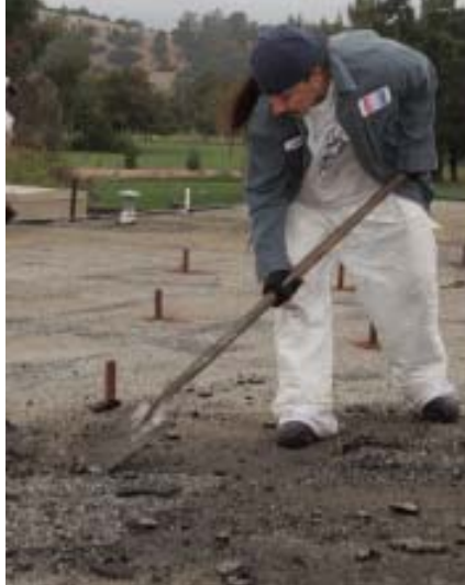
Figure 2. To prep the roof, workers sweep up and remove loose aggregate (above left) and scrape up poorly bonded areas of asphalt and gravel (above right). Once the roof is clean, they spray on a primer to make the foam stick better (right). The vertical posts — which were just installed — will be used to support solar panels.
