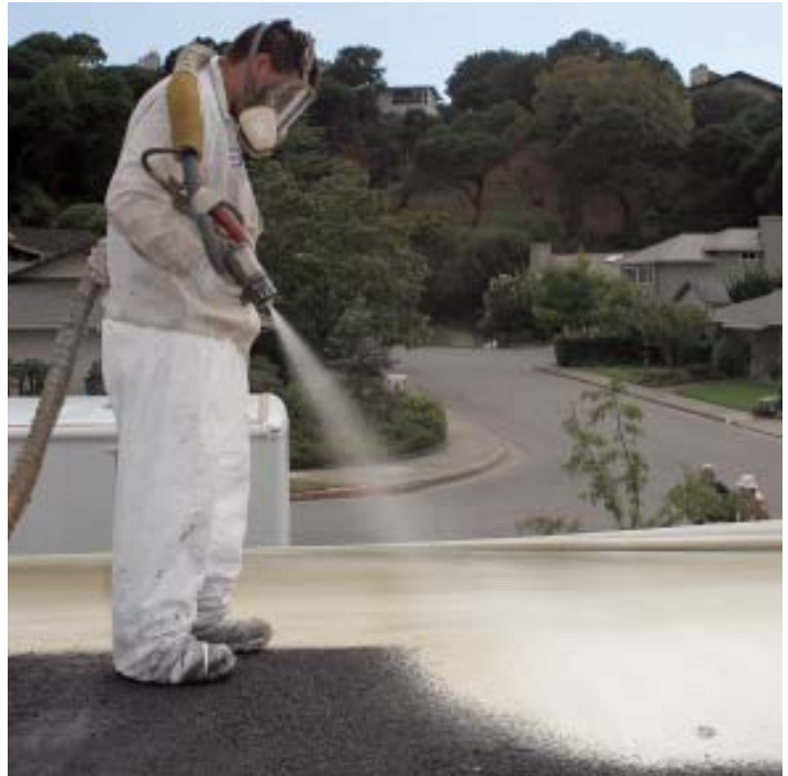
Figure 7. The applicator pulls up on the masking paper while spraying foam up and onto the edge metal (above left). After spraying such detail areas as edges, curbs, and roof jacks, he sprays the main body of the roof (above). A worker uses a grinder to bring the foam flush to the edge metal (left) and to make it slope properly into scuppers and drains.
