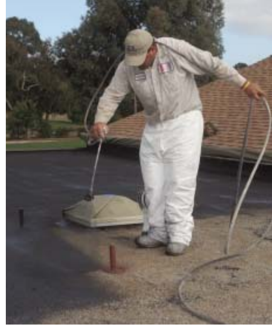
Figure 2. To prep the roof, workers sweep up and remove loose aggregate (above left) and scrape up poorly bonded areas of asphalt and gravel (above right). Once the roof is clean, they spray on a primer to make the foam stick better (right). The vertical posts — which were just installed — will be used to support solar panels.
