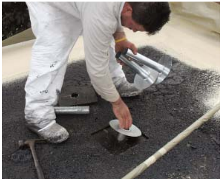
Figure 4. Although some sheet metal can be reused, scuppers (above) and drains should be replaced so the foam has a clean surface to bond to. Here, a roofer cuts out the membrane around an existing drain (above right); it's replaced with a new dropout fitting (right) that feeds to a downspout below. The new fitting will be nailed to the deck and primed before the foam is applied.
