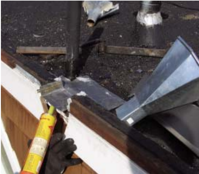
Figure 4. Although some sheet metal can be reused, scuppers (above) and drains should be replaced so the foam has a clean surface to bond to. Here, a roofer cuts out the membrane around an existing drain (above right); it's replaced with a new dropout fitting (right) that feeds to a downspout below. The new fitting will be nailed to the deck and primed before the foam is applied.
