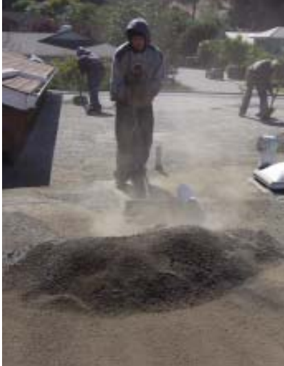
Figure 2. To prep the roof, workers sweep up and remove loose aggregate (above left) and scrape up poorly bonded areas of asphalt and gravel (above right). Once the roof is clean, they spray on a primer to make the foam stick better (right). The vertical posts — which were just installed — will be used to support solar panels.
