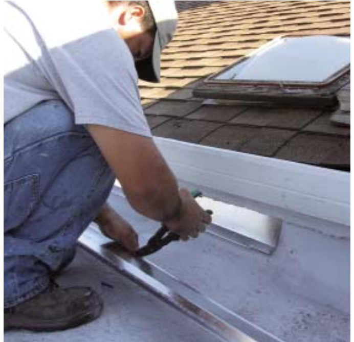
Figure 5. Foam is self-flashing when applied to waterproof substrates, but water can still get behind wall cladding. Therefore, the crew breaks out this stucco, slips counterflashing behind the building paper, and laps it over the foam below (above). Where the foam runs up onto the wall, the roofer laps over it with flashing that tucks behind the gutter (right).
