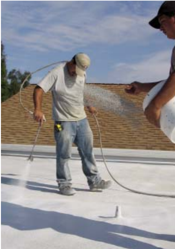
Figure 8. To prevent UV rays from degrading the foam, the crew coats the surface with a protective elastomeric coating. The base coat goes on first and dries overnight. Then the top coat is applied; while it's still wet, a worker broadcasts a layer of mineral granules onto it (left). The finished roof (above) is a monolithic waterproof membrane with an R-value of about R-6.5 per inch of thickness.
