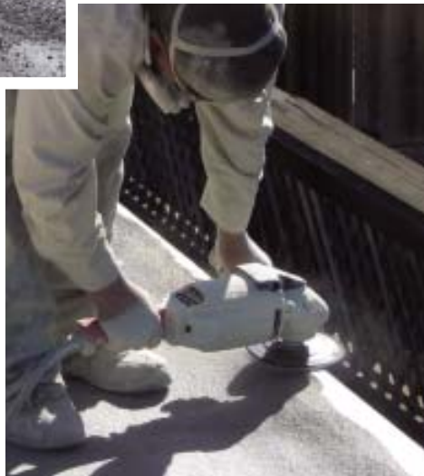
Figure 7. The applicator pulls up on the masking paper while spraying foam up and onto the edge metal (above left). After spraying such detail areas as edges, curbs, and roof jacks, he sprays the main body of the roof (above). A worker uses a grinder to bring the foam flush to the edge metal (left) and to make it slope properly into scuppers and drains.
