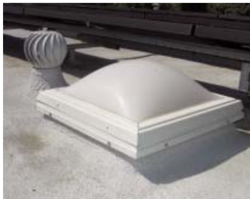
Figure 6. The crew takes skylights off the curbs before applying foam. This curb will be too close to the surface after the foam is applied, so the roofers extend it with a wood frame (above left). Then they mask the opening and waterproof it with a layer of foam (above). Once the rest of the roof has been foamed and coated, they remove the masking, apply weather-stripping to the curb top, and reinstall the skylight (left).
