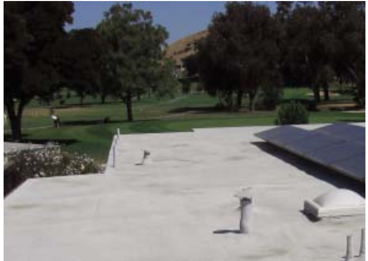
Figure 8. To prevent UV rays from degrading the foam, the crew coats the surface with a protective elastomeric coating. The base coat goes on first and dries overnight. Then the top coat is applied; while it's still wet, a worker broadcasts a layer of mineral granules onto it (left). The finished roof (above) is a monolithic waterproof membrane with an R-value of about R-6.5 per inch of thickness.
