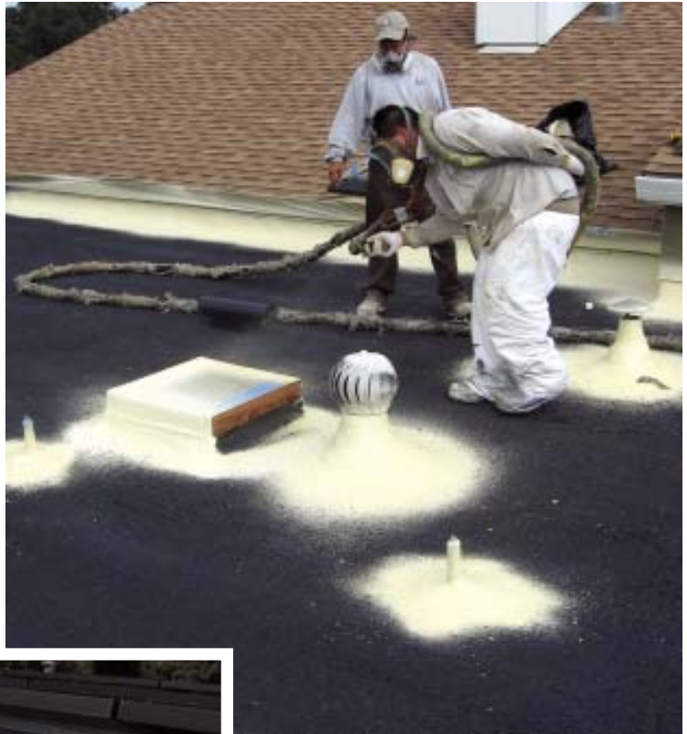
Figure 6. The crew takes skylights off the curbs before applying foam. This curb will be too close to the surface after the foam is applied, so the roofers extend it with a wood frame (above left). Then they mask the opening and waterproof it with a layer of foam (above). Once the rest of the roof has been foamed and coated, they remove the masking, apply weather-stripping to the curb top, and reinstall the skylight (left).
