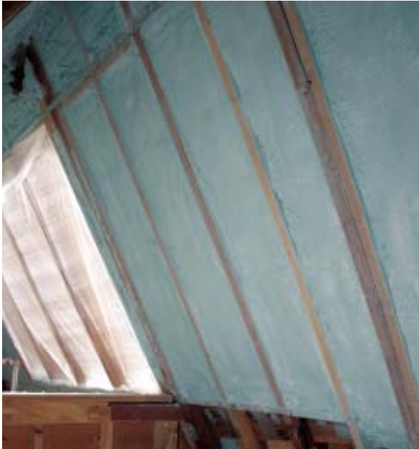
Figure 5. Open-cell foam, which expands to about 100 times its liquid volume, typically has to be trimmed flush to framing members — an easy task, since the foam is so soft. Because of its lower expansion rate and higher R-value per inch, closed-cell foam doesn't usually have to be trimmed. When it does, as in this shallow rafter bay (left), the author's crew uses a scraper — in this case a horse curry comb — to clean the framing in preparation for drywall (right).
