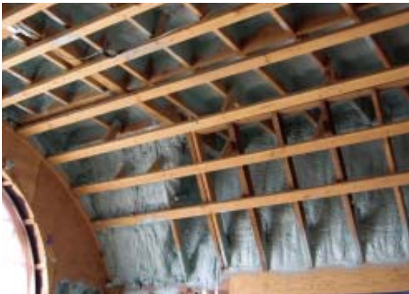
Figure 4. This barrel ceiling (above) would be difficult to insulate and seal with traditional materials. It's an ideal candidate for spray foam, which conforms to its irregular surfaces (left).
